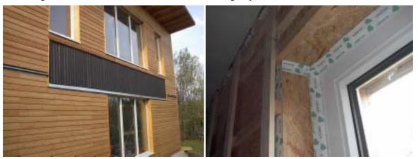
A pioneering project which developed a 'puzzle system' for assembling the house's raw construction from six pieces (floor, four walls and roof) for the price of a regular prefabricated house, plus the quality of a passive house. The visible material of the house is wood, which was used also for the load-bearing elements. The main component of the walls are straw bales. The picture shows a close-up of the insulation of the interior panelling of the house.
