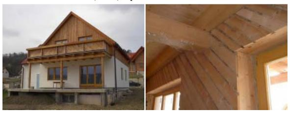
The house in Breitenfeld violates the principles of the passive house a little bit; the builder decided to use cheaper windows. What is interesting, though, is the construction, in which straw bales were pressed into the wooden frame. Straw insulates as well as styrofoam, but is much cheaper and nobody needs to worry about waste. On the contrary; the more straw is deposited within the walls, the better, as the straw stores carbon dioxide taken from the air.
